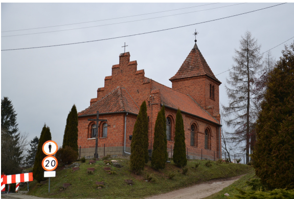
Fig. 4. Church in Bukwałd – a positive example of the region's countryside architecture
